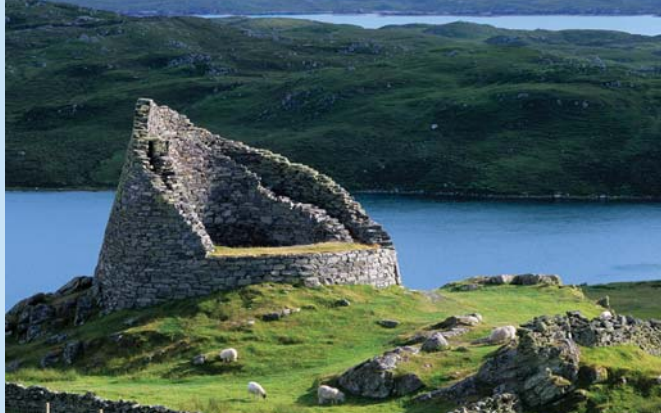
Dun Carloway is just one of Scotland's Iron-Age brochs, impressive circular towers representing the pinnacle of drystone construction.
