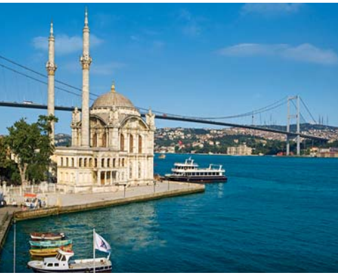
The spectacular Bosphorus Bridge in Istanbul spans between the two continents of Europe and Asia.
