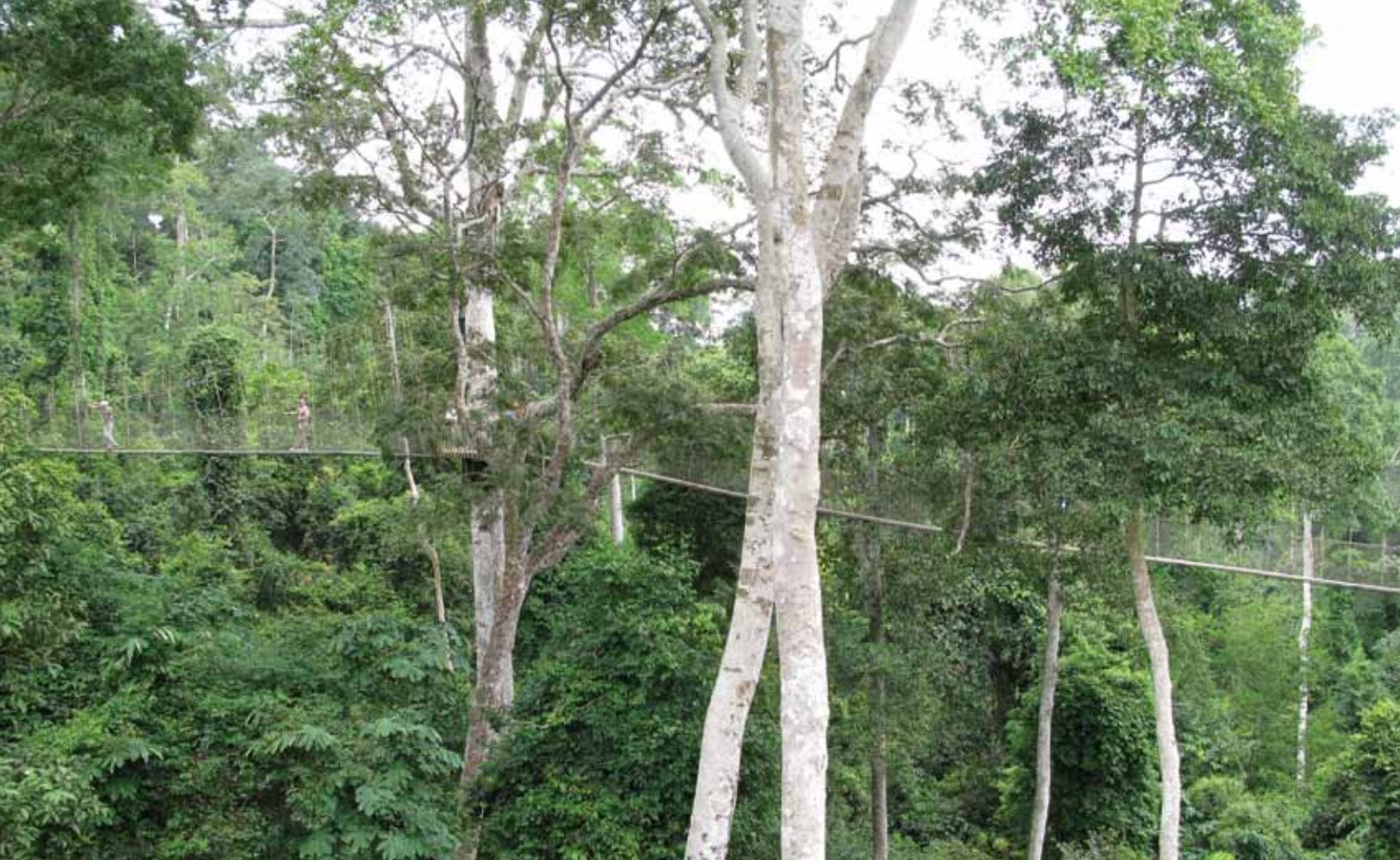
Kakum National Park's aerial walkway soars above the floor of the rain forest in Ghana
